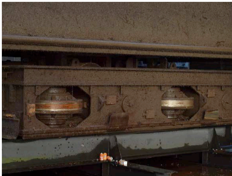
Figure 9 Lower roller carriage with two of the guiding wheels visible (source: Rijkswaterstaat)
